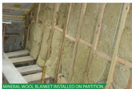
MINERAL WOOL BLANKET INSTALLED ON PARTITION
