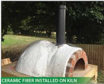
CERAMIC FIBER INSTALLED ON KILN
