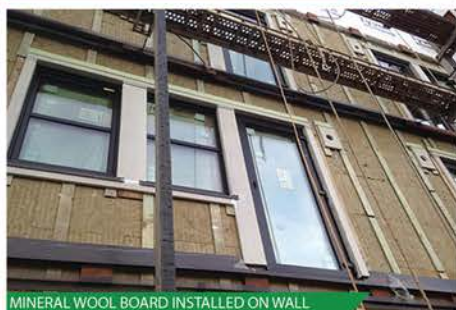
MINERAL WOOL BOARD INSTALLED ON WALL
